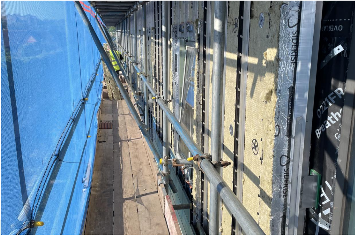
Installation Of Rails & Insulation
