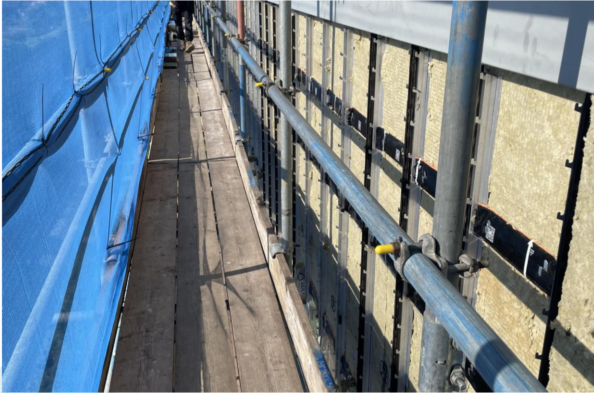
Installation of Rails/Fire Barrier & Insulation
